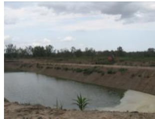
7. New pond approximately 50 x 20 m x 5 m – one of five new ponds; part-filled with irrigation water.
