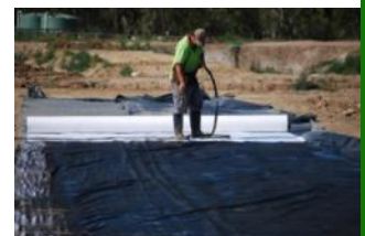
12. Liquid Rubber being sprayed on geofabric.
