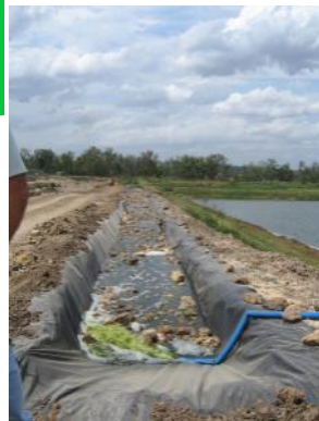
4. Longitudinal view of riffle bed – approximately 120m long. The flow is to increase to over 10L/s to create a more turbulent flow. Note the heavy algal growth.
