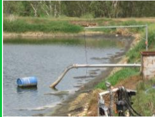
3. Number 3 Aerobic Lagoon – note sludge that is accumulating around the edges of the pond due to overloading.
